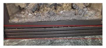
**STEP 2:** The manufacturer, model and serial numbers are located on a "rating plate," which is a metal plate that is usually permanently affixed to the fireplace. The rating plate will be located on the bottom left or right side of the fireplace.
